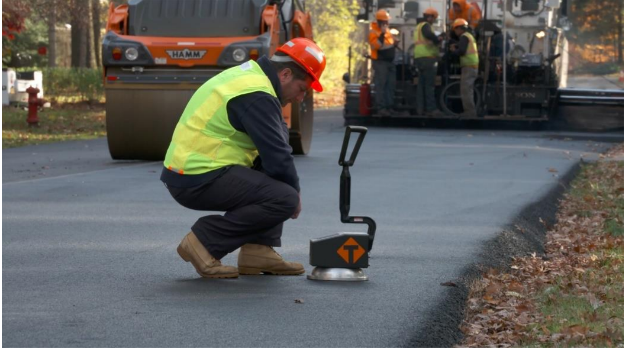
Figure 1: Checking asphalt density with a non-nuclear, non-destructive method
